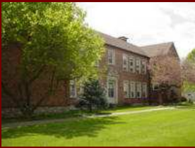
Benton Elementary School, One of five Columbia schools recognized for superior energy performance.
